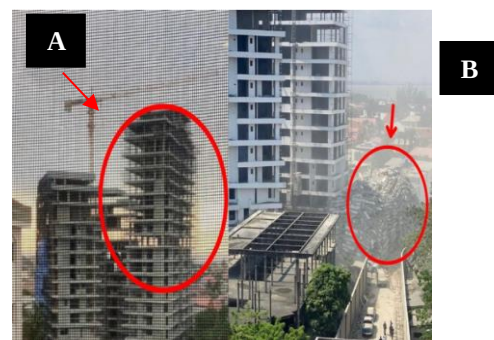
Figure 3. 21-Story Building Collapse in Lagos State
